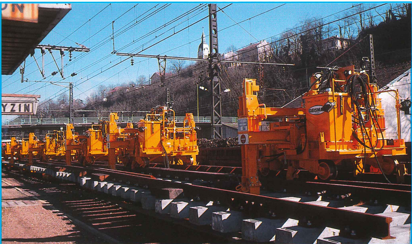
Laying of a concrete sleepers turnout of 45 metres (55 t).
