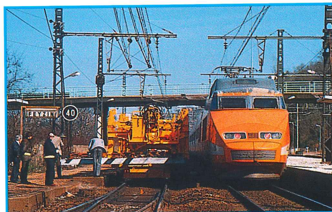
Worksite on double track with traffic on adjacent line.
