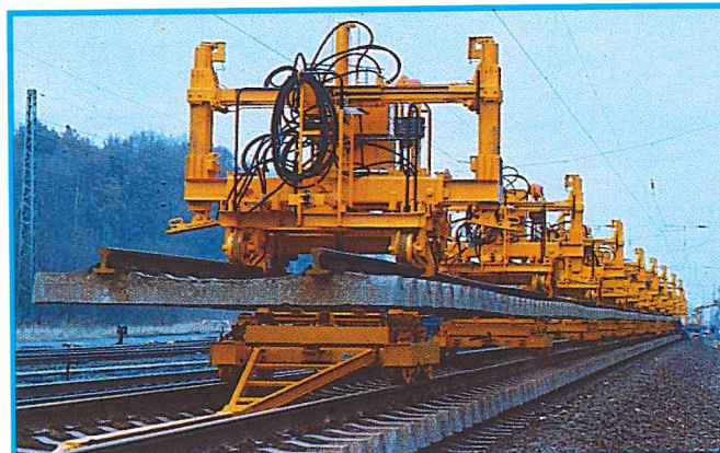
180 m track panel laying with concrete sleepers (100 t).
