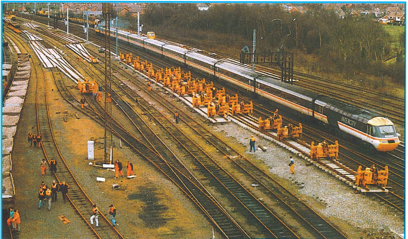
Laying of a concrete sleepers prefabricated crossover of 150 metres (200 t).
