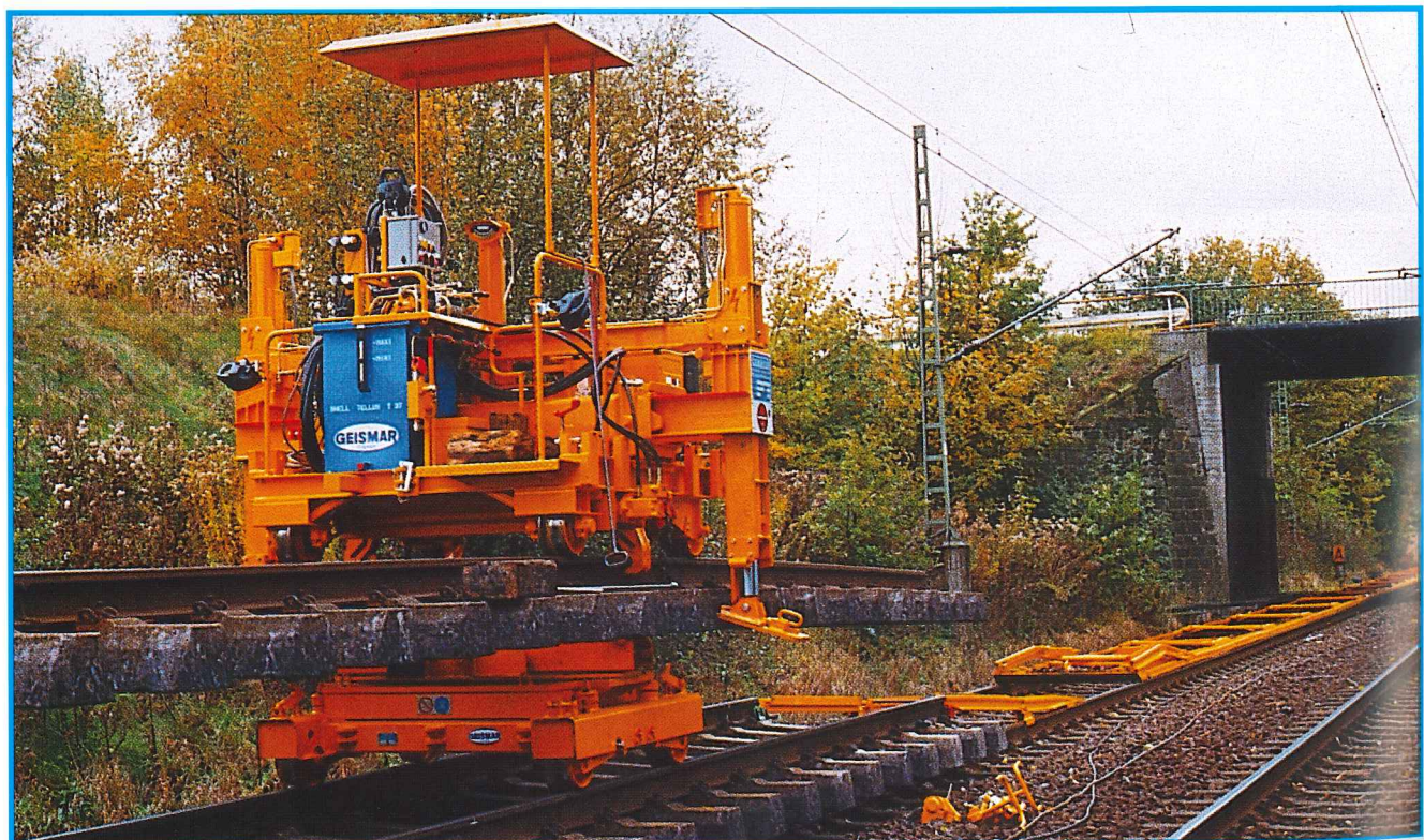
Reballasting and reblanketing works
